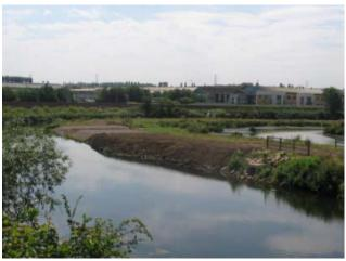
**Solution:** Filtrexx Soxx and Coir Matt were installed along the riverbank in 20m sections. The Filtrexx was filled with locally sourced PAS100 compost and a mix of wetland seeds native to the local area. The Soxx withstand any erosion and retain the compost allowing seeds the opportunity to germinate. The roots of these wetland plants soon take hold and reinstate the banking. The soxx were installed and staked directly onto the banking.
